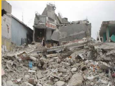
The local pediatrics clinic was destroyed by the earthquake.
